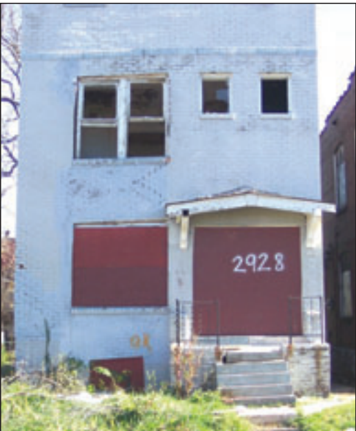
A future building to be refurbished.
