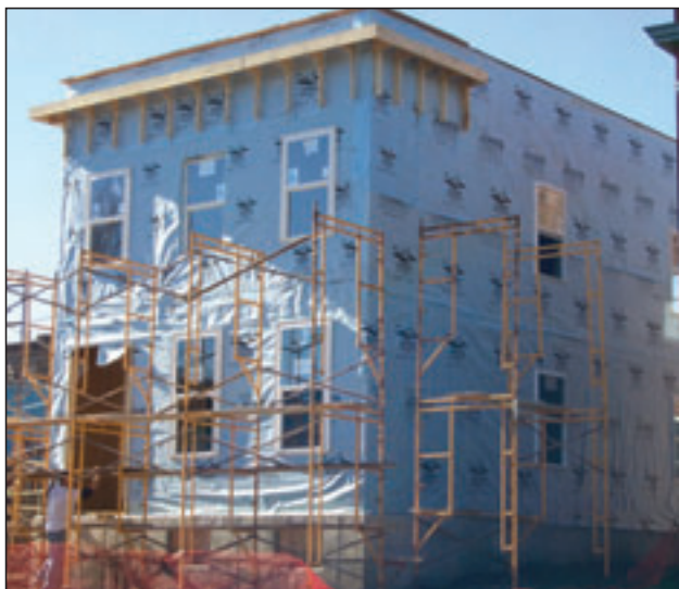
A Benton Park West Corp. home with renovations in process.
