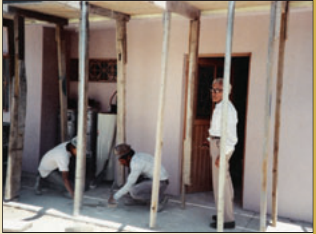
The Convent under construction.
